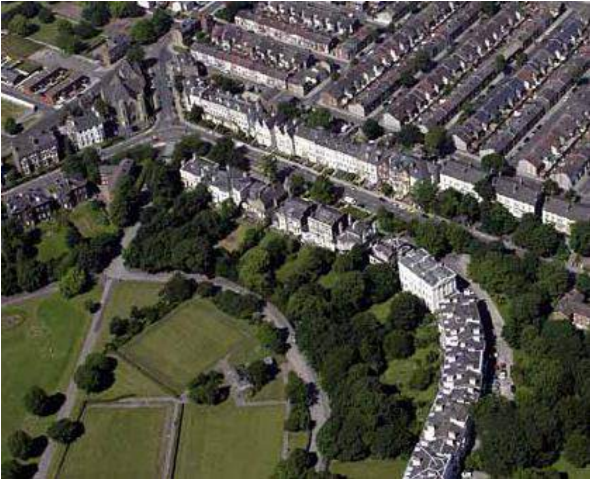
The north end of Joseph Paxton's GII* listed Princes Park, showing the proximity and intimate relationship of the 1870s Welsh Streets terraces to the listed villas of the conservation area round the park.
