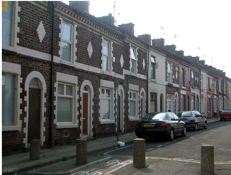
Above: Vienna Street, Anfield, 2007. Demolished 2014.
